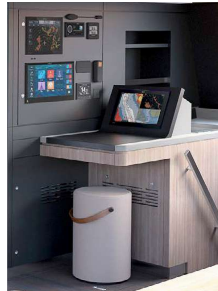
A dedicated chart table is discretely placed but bursting with technical capabilities
